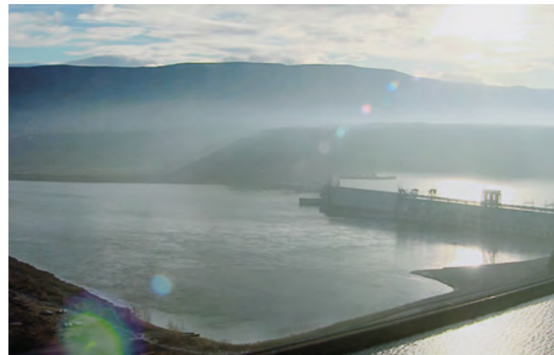
Using renewable energies: hydropower plants on the Columbia River supply the Moses Lake facility.
