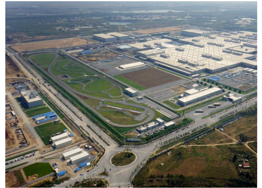
REDUCING USE OF DRINKING WATER AT PRODUCTION PLANTS — BMW Brilliance Automotive plant in Tiexi (China)
