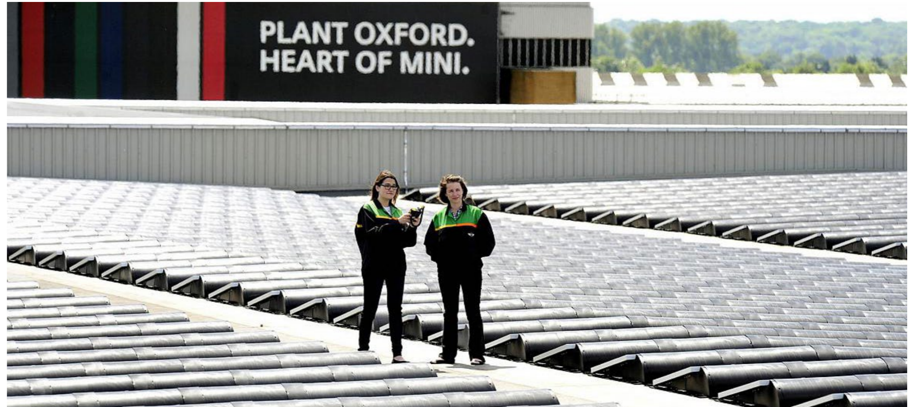
RENEWABLE ENERGY FOR PRODUCTION OF THE MINI — Solar panel system at the plant in Oxford (UK)
