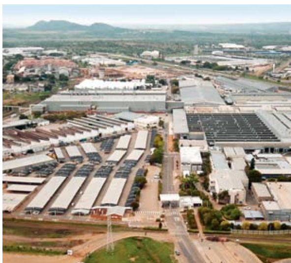
BMW PLANT ROSSLYN — Plans for a twin-unit power station fuelled by landfill gas.
