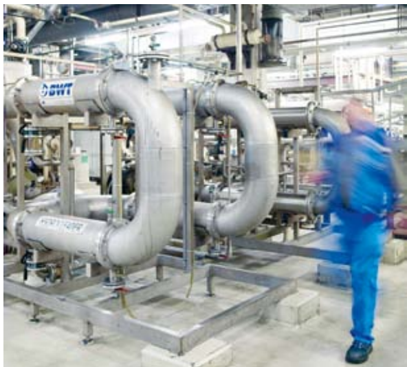
BMW PLANT STEYR — Electricity generated from biomass.
